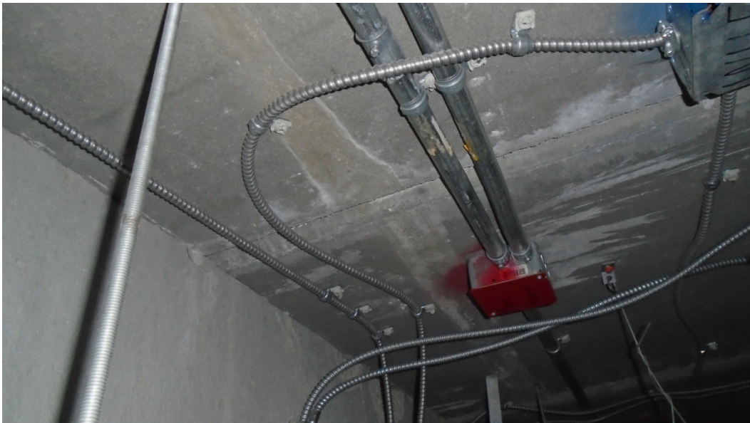
Photo 34: Concrete wall support of perpendicular hollow core planks floor system on east side of grid 5. Wall is supporting the 2 nd floor structural hollow core plank floor system as seen from ceiling.
