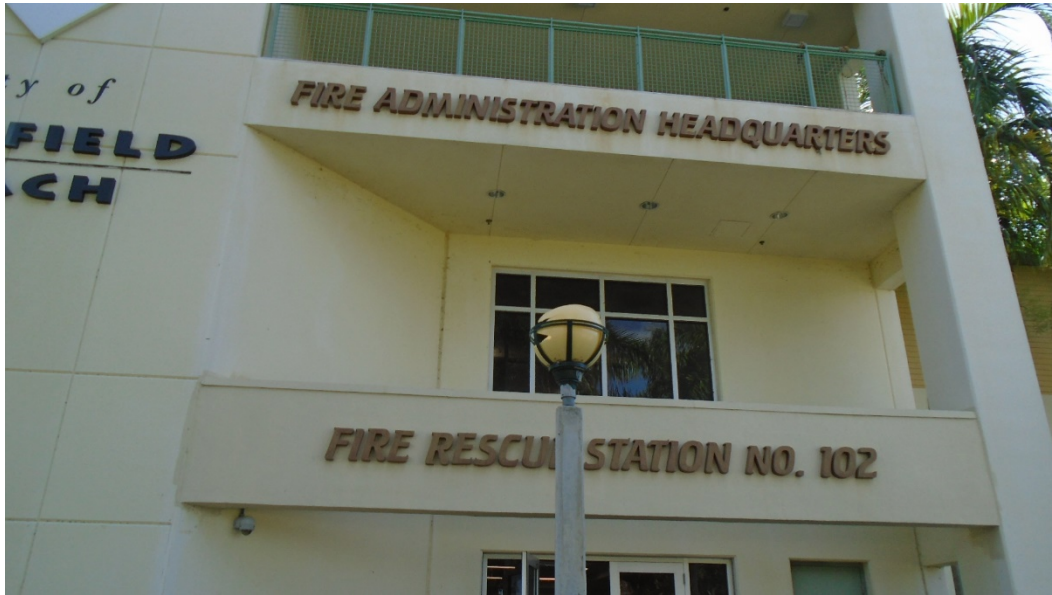
Photo 1: West side entrance general building condition.
