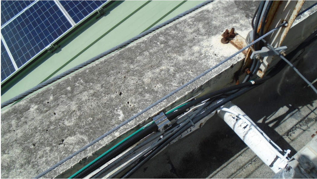
Photo 38: Above stair#2, exposed concrete at parapet walls in roof area 3 per Advance Roofing Report.
