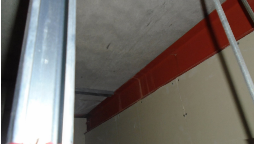
Photo 33: Steel channel ledge support of parallel hollow core planks floor system on west side of grid 5. Steel channel is supporting the 2 nd floor structural hollow core plank floor system as seen from ceiling.
