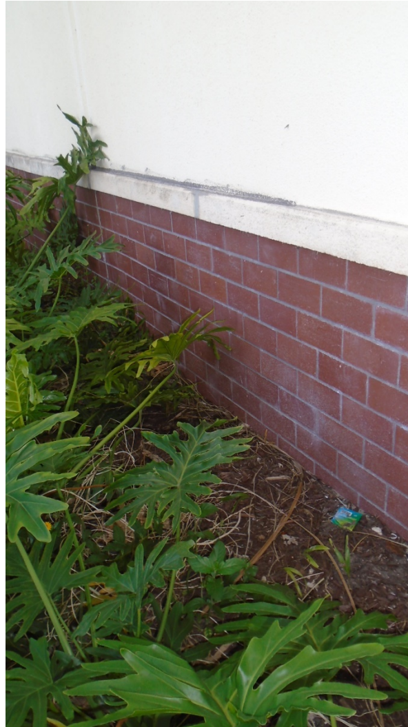
Photo 19: Existing decorative 4" split face brick veneer found throughout the lower portion of building.
