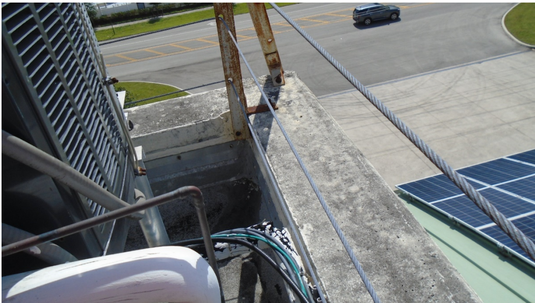
Photo 39: Above stair#2, exposed concrete at parapet walls in roof area 3 per Advance Roofing Report.
