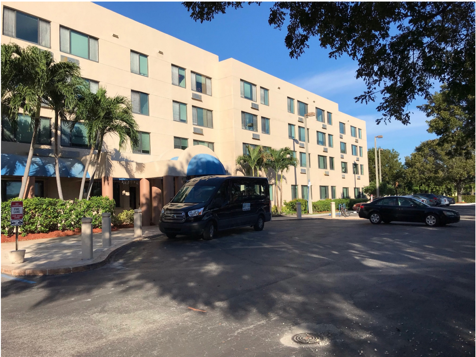
North-West View – Main Entrance
