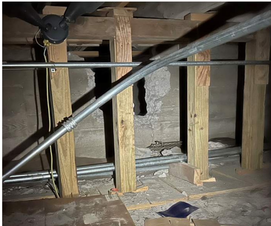
Photo 17 – Added support for framing at the auditorium stage
