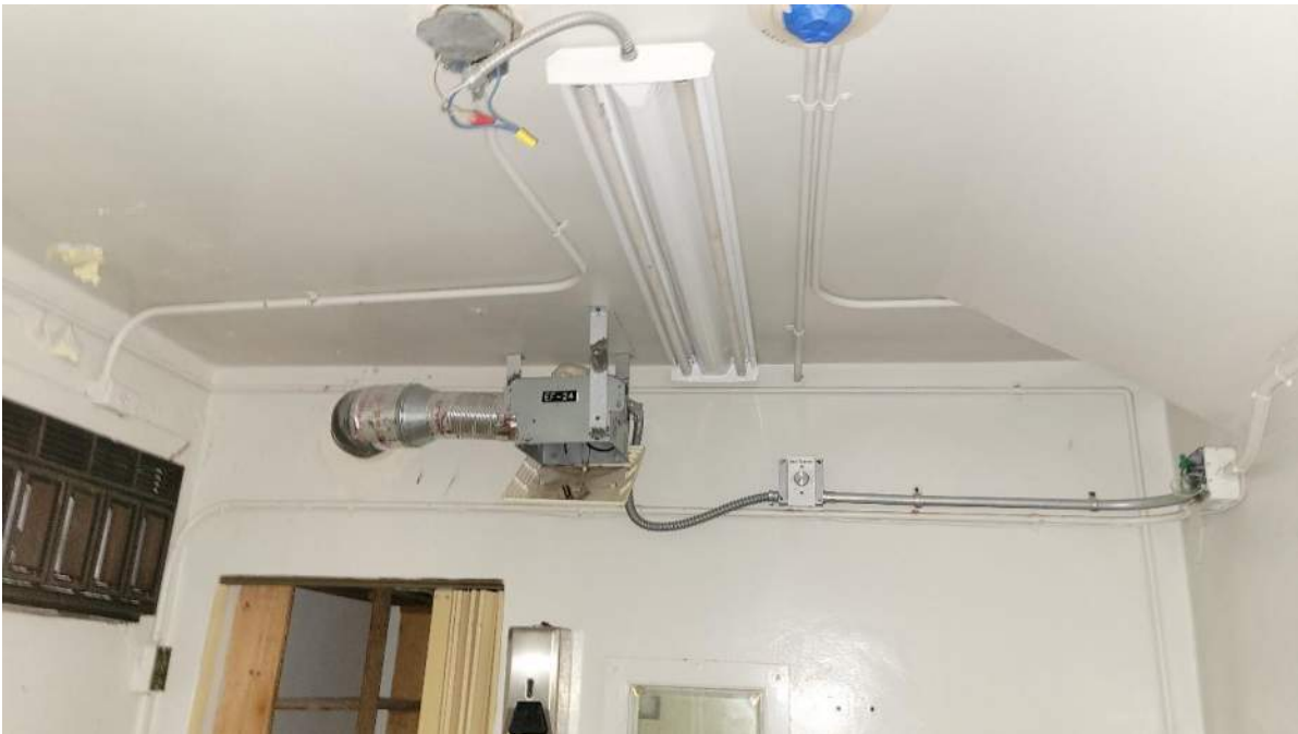
Rm. 106a – Ceiling of existing restroom
