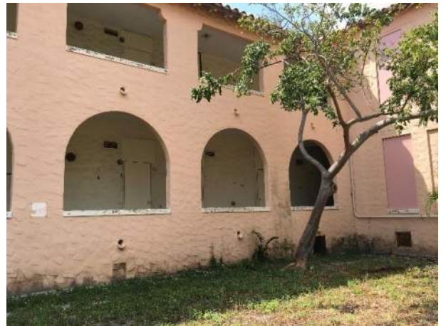
Northwest Corner of East Wing
