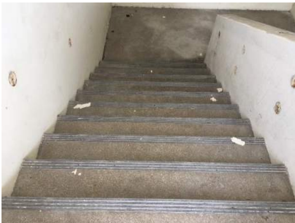
North Stair at West Wing Upper Landing
