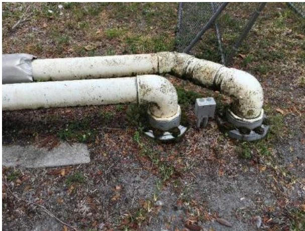
Exterior – Outside of Boiler Room
