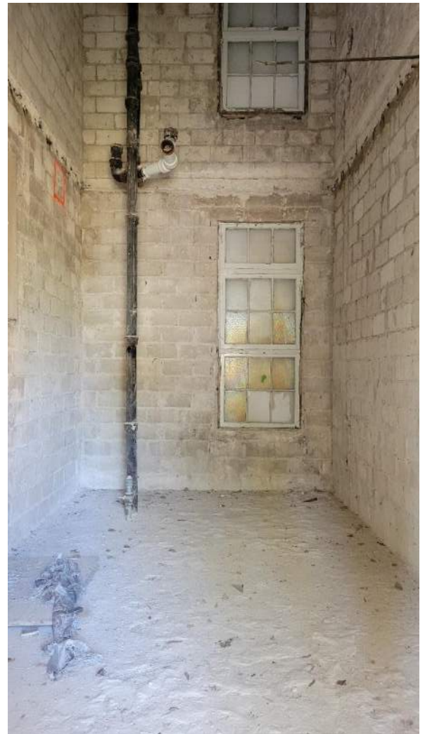
Room 111 – RWL location off East wall to be addressed. Second floor slab removed; to be replaced with new floor
