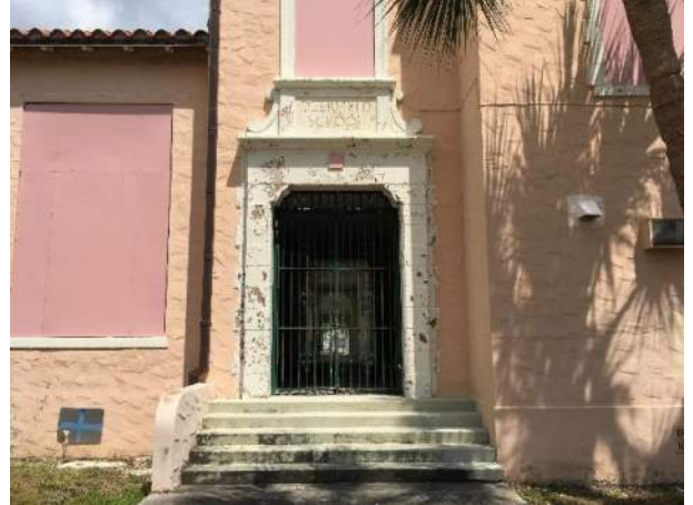
Front Entrance – South Elevation
