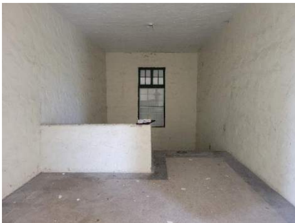
South Stair at 2 nd Level
