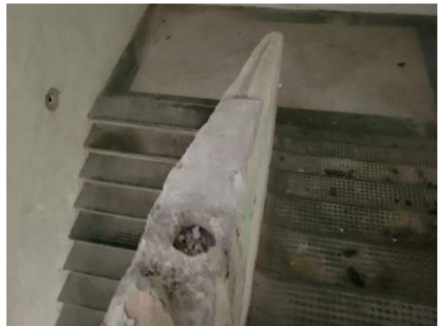
South Stair – Railing Removed
