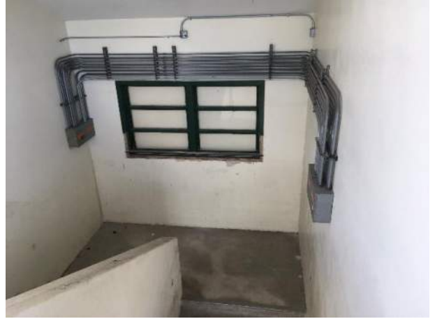
North Stair at West Wing – 2 nd Level
