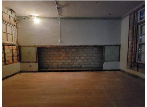
Room 125 – Void left by existing casework
