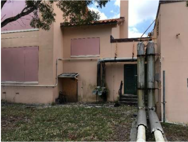
Exterior – Outside of Boiler Room
