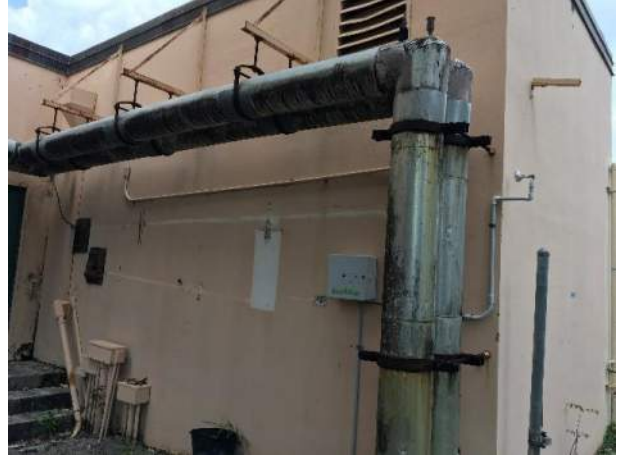
Exterior – Outside of Boiler Room
