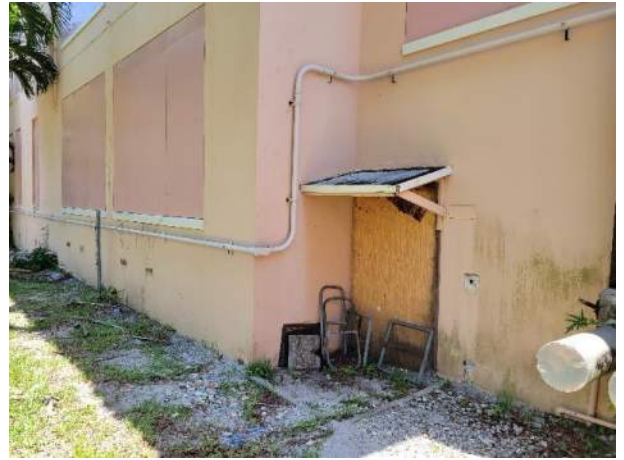
Exterior – Outside of Room 116 – Not in use (No Access)
