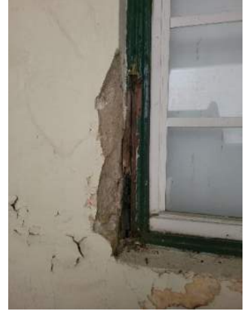
Window at South Stair
