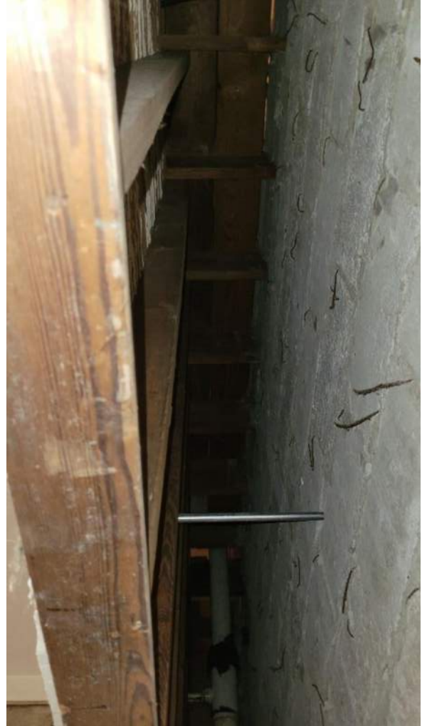
Room 110 – View inside of Chase in room
