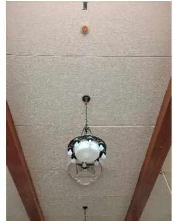
Rm. 101 - Ceiling at lights in Auditorium
