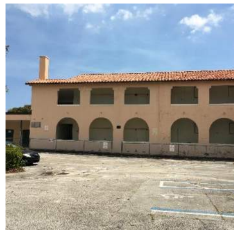
West Elevation of North Wing
