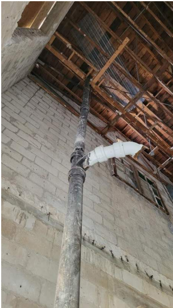
Room 111 – RWL location off North wall to be addressed. Second floor slab removed; to be replaced with new floor
