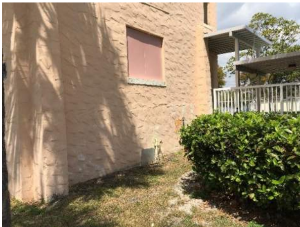
East Elevation of East Wing
