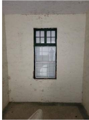
Window at South Stair
