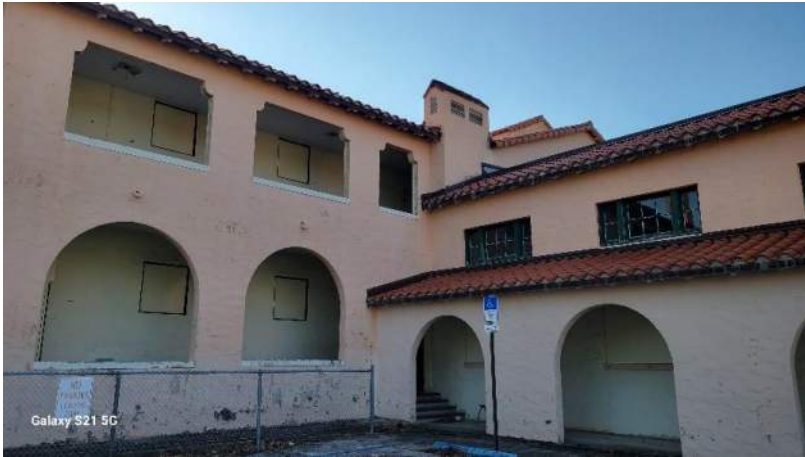
Southwest Corner of North Wing
