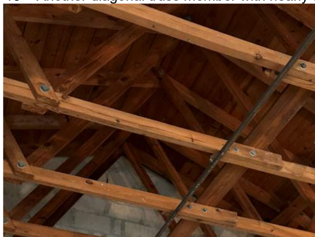
Photo 16 – Wood truss framing at the 1954 classroom addition
