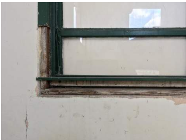
North Stair at West Wing Window Sill
