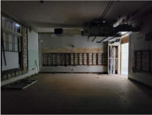
Room 122 – Chase in room at classroom entrance
