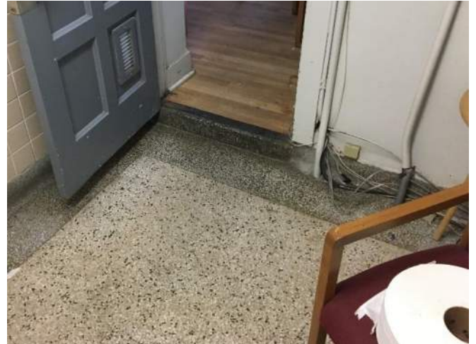
Rm. 106a – Flooring height difference (shown for reference)
