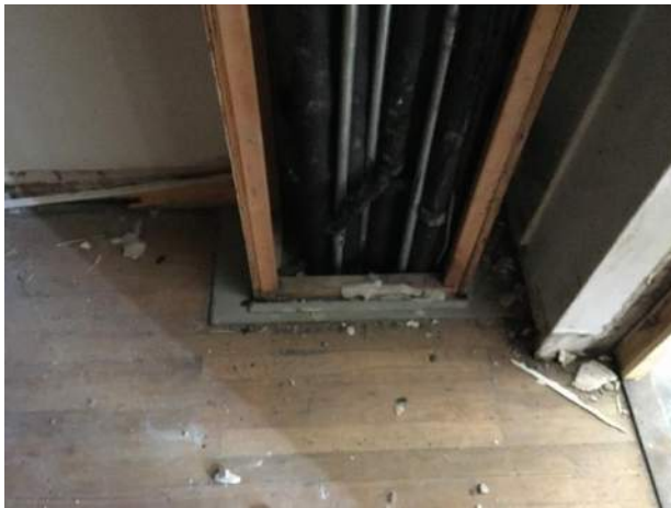
Room 125 – Chase in room
