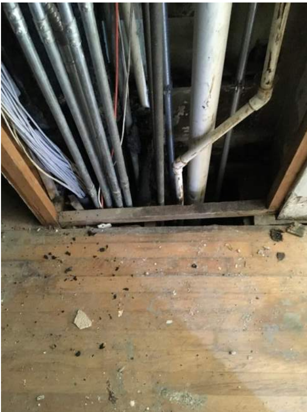
Room 122 – Chase in room
