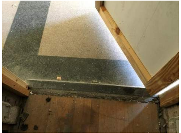
Room 122 – Classroom entrance
