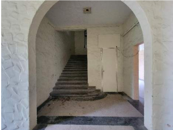
South stair at ground Level
