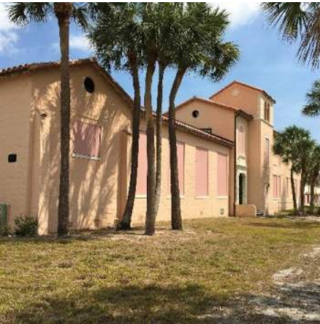
South Elevation of West Auditorium Wing
