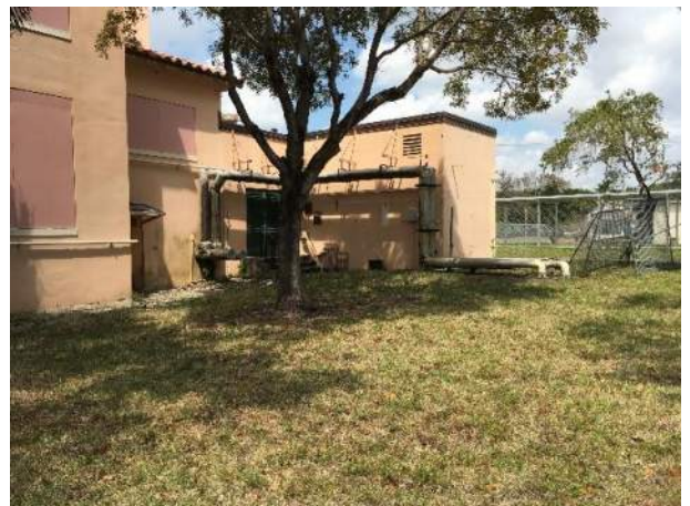
Northeast Corner of North Wing
