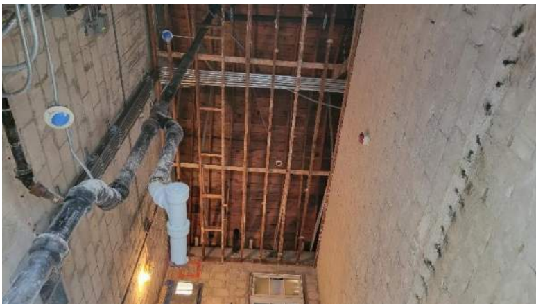
Room 113 – Existing electrical conduits. Second floor slab removed; to be replaced with new floor
