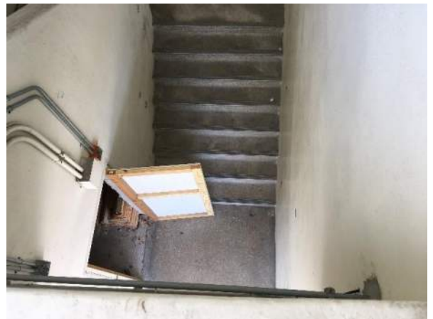
North Stair at West Wing
