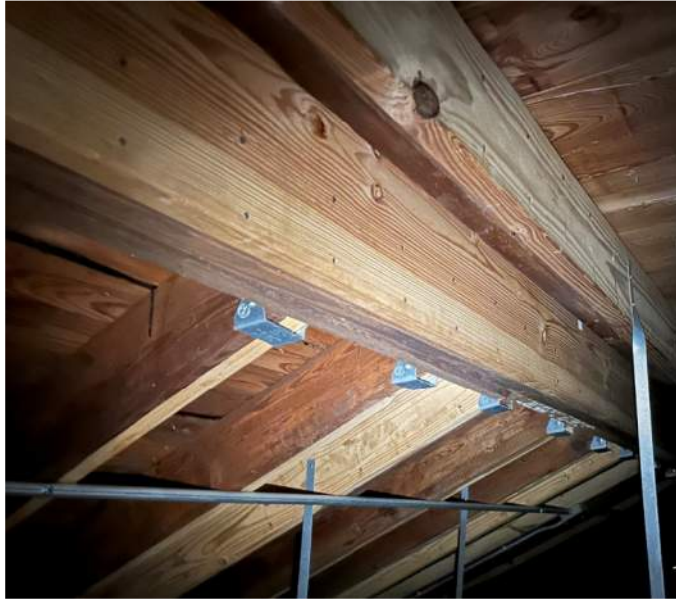
Photo 1 -Doubled up roof framing at Auditorium Attic
