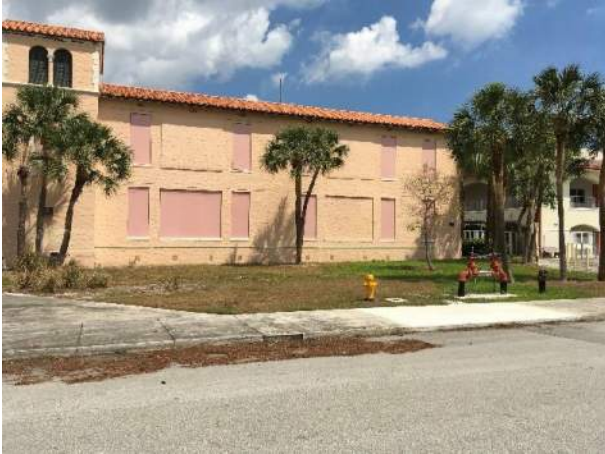
South Elevation of East Wing
