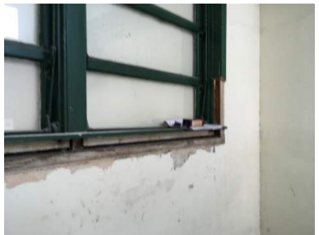
North Stair at West Wing Window Sill
