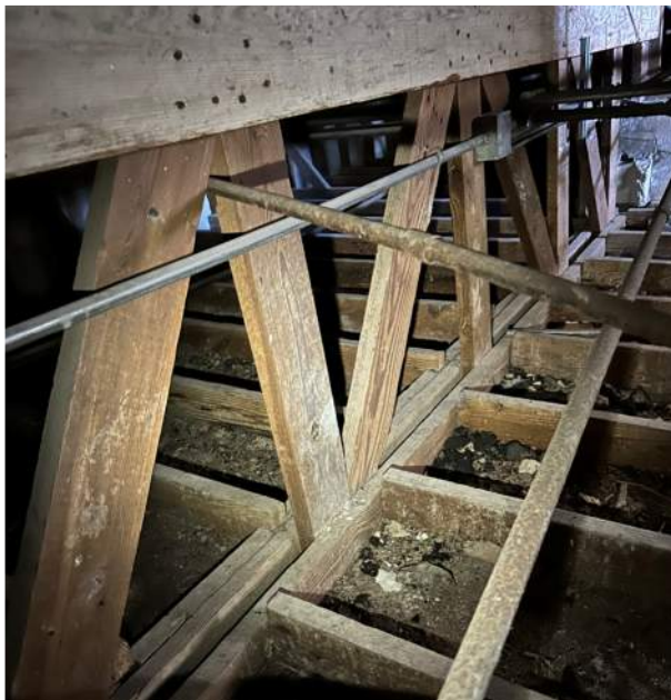
Photo 4 – Ceiling Framing with Wood Truss above stairs.
