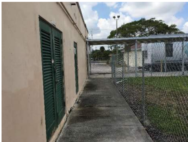
View of North Elevation of North Wing
