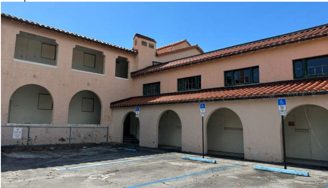
Photo 26 – Northwest side of the building showing the exterior concrete walls with arches
