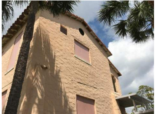
East Elevation of East Wing
