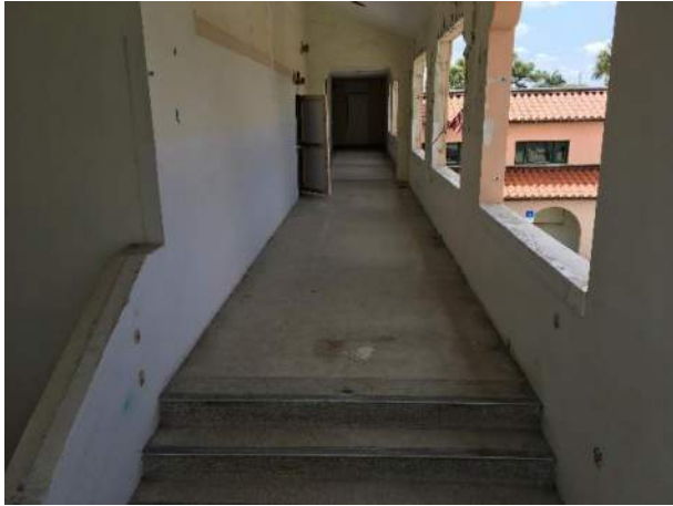
North Stair at West Wing – 2 nd Level
