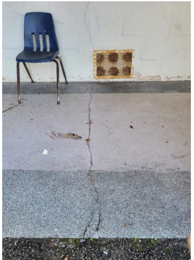
Exterior Flooring Condition – Outdoor corridor North of Auditorium
