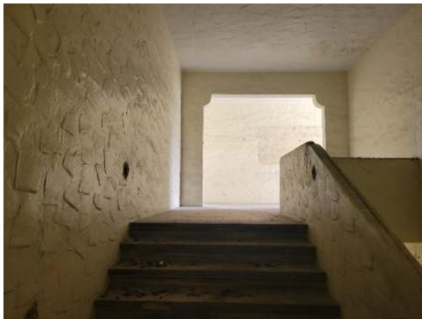
South Stair - Upper Landing
