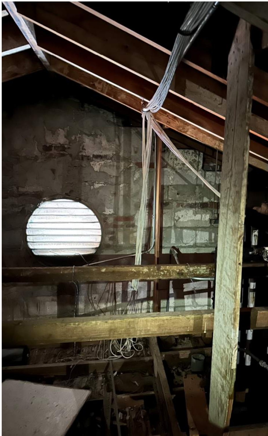
Photo 11 – Wood hangers from roof rafters support ceiling beam
