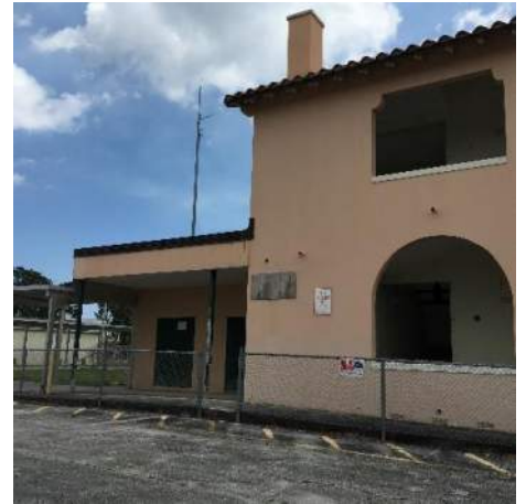
Northwest Corner of North Wing
