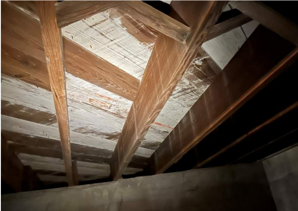
Photo 20 – Wood framing under east wing classroom
