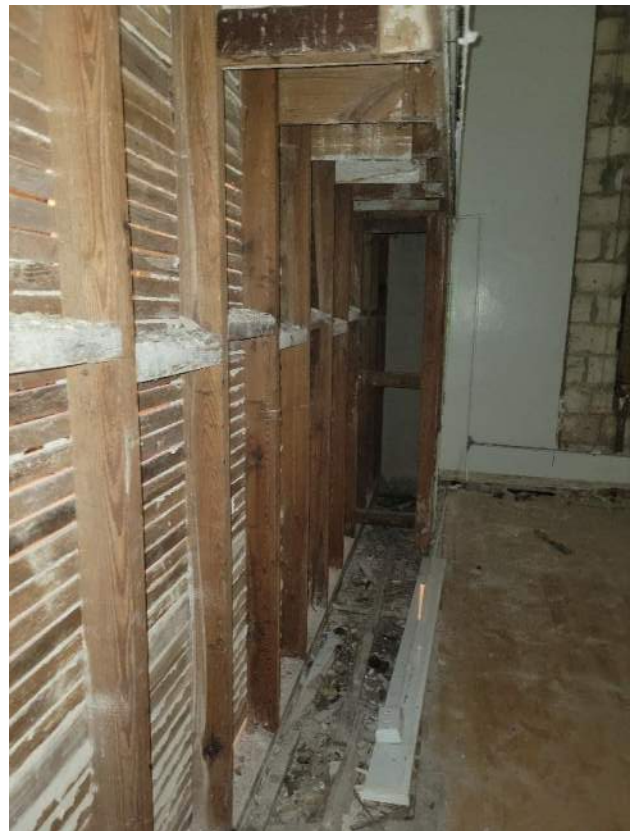
Room 122 – Void left by existing casework
