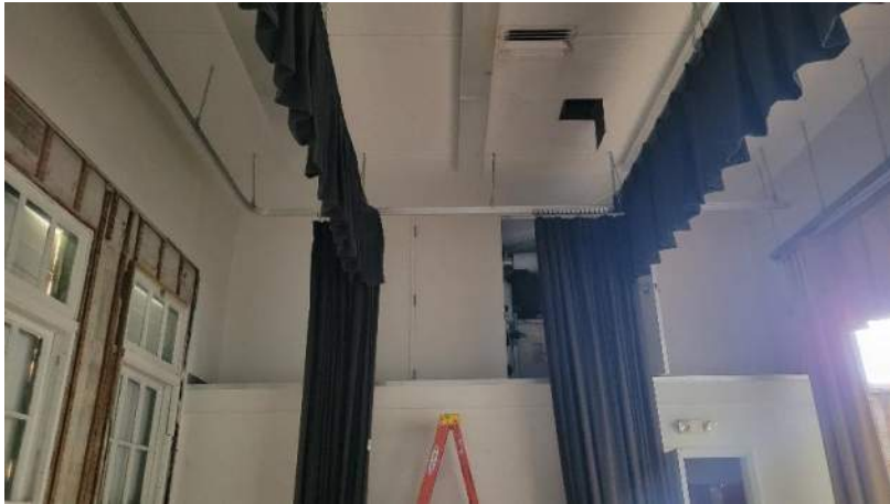
Rm. 101A - Mechanical Mezzanine Above Stage storage spaces
