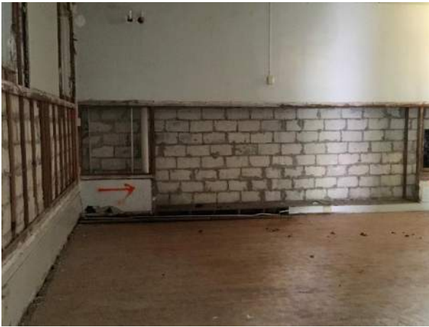
Room 123 – Void left by existing casework
