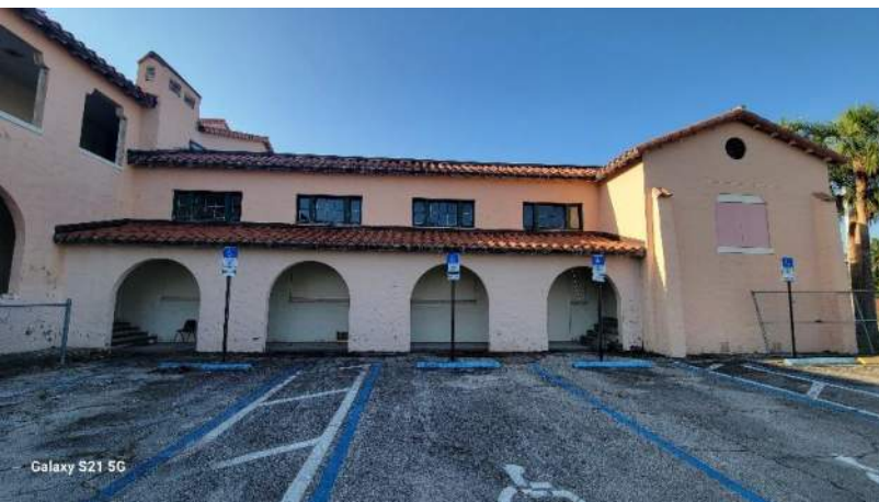
North Elevation of West Wing
