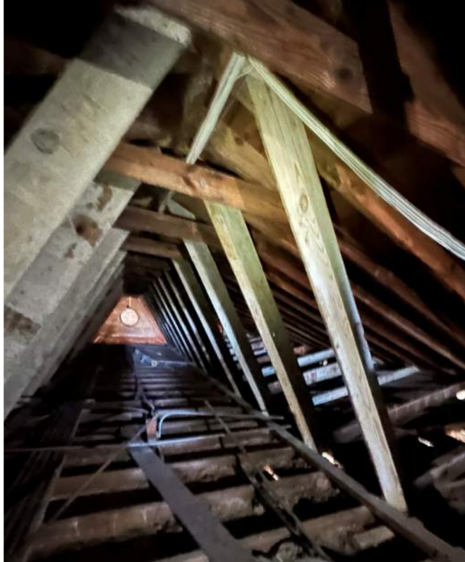
Photo 12 -Alternate truss & "collar-tied" roof rafter framing
