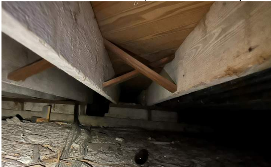
Photo 19 – Auditorium floor framing from crawl space
