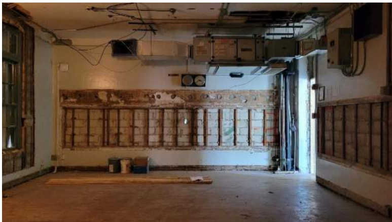
Room 112 – Chase in room
