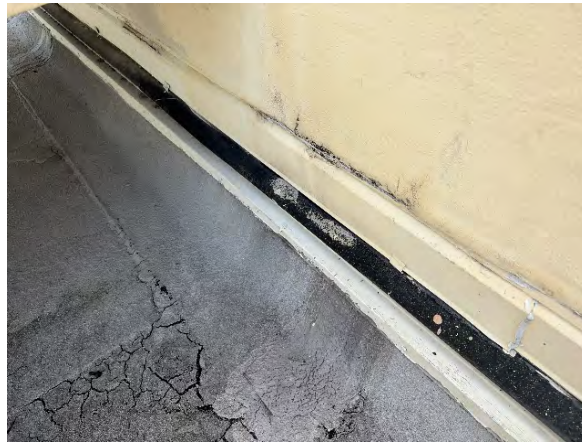
Typical expansion joint
