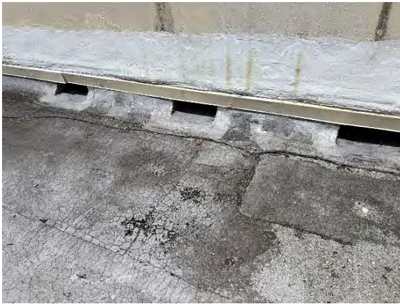
Typical primary scupper with flashing detail
