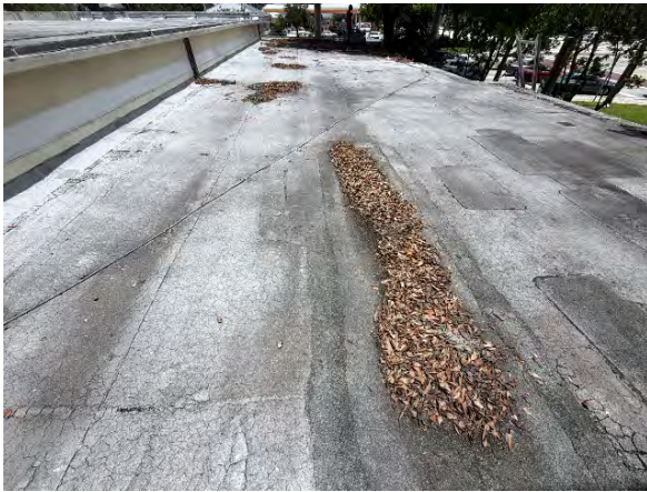
Roof overview facing north
