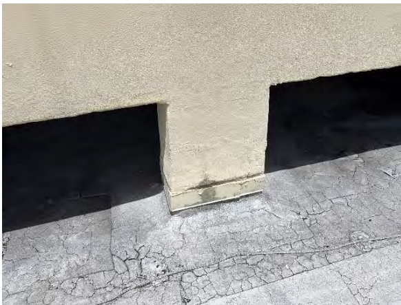
Column support with base flashing detail
