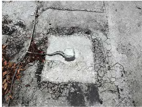
Typical pitch pan flashing detail
