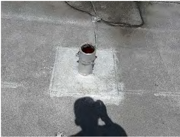
Typical plumbing stack with flashing detail
