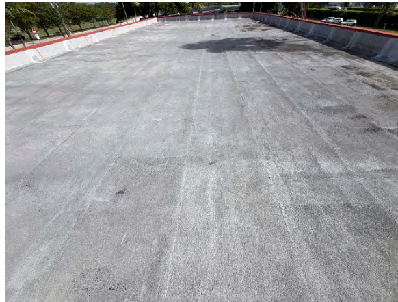
Roof overview facing north
