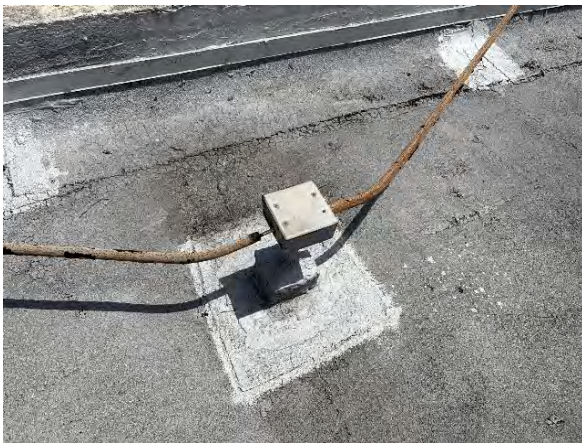
Typical pitch pan flashing detail
