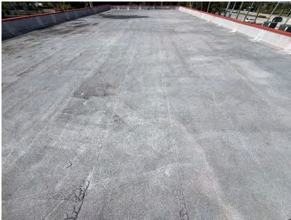
Roof overview facing south
