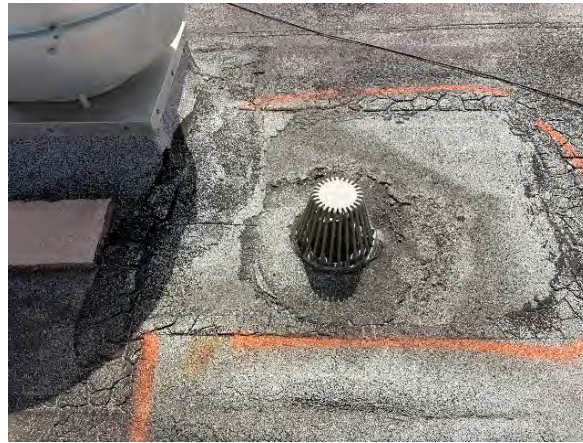
Typical retrofit with flashing detail
