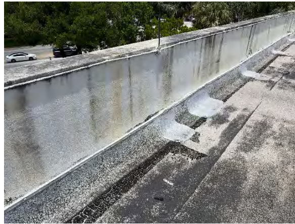
Typical parapet wall with base flashing detail
