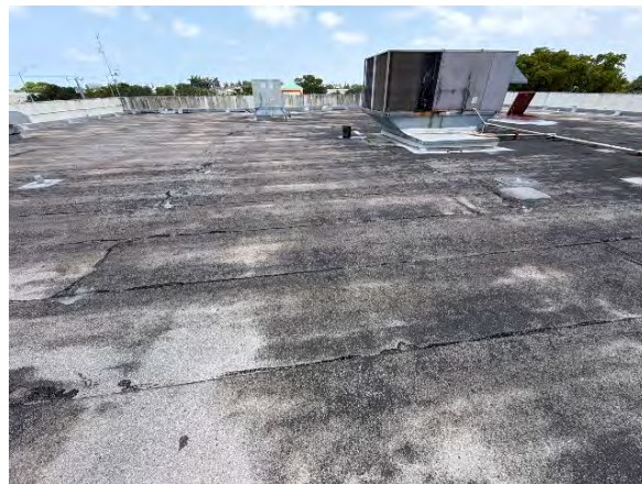
Roof overview facing south
