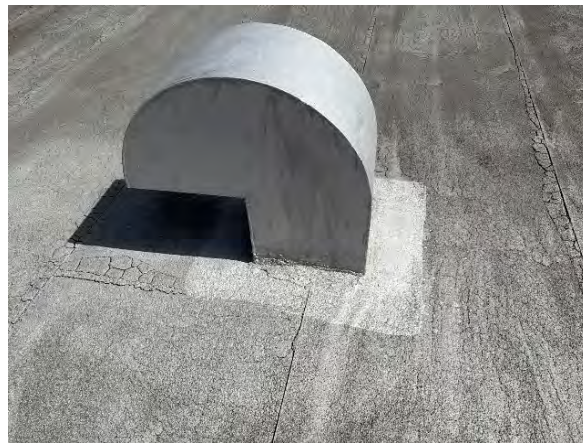
Typical gooseneck with flashing detail
