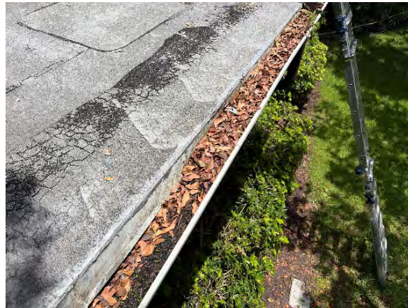
Typical gutter system with downspouts
