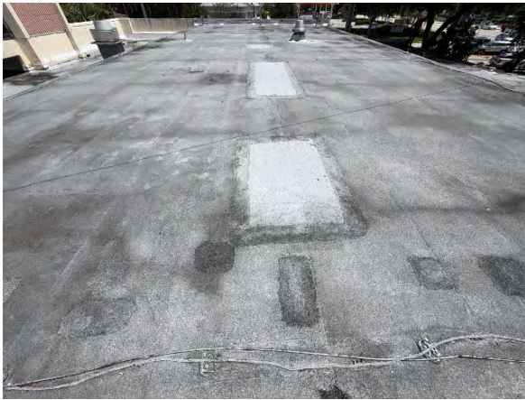
Roof overview facing north
