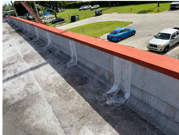
Typical parapet wall with base flashing detail
