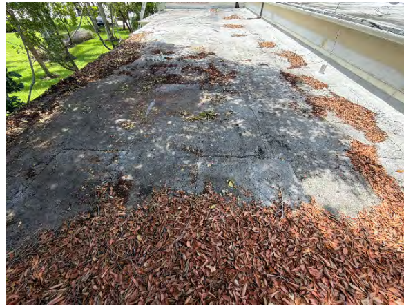
Roof overview facing south
