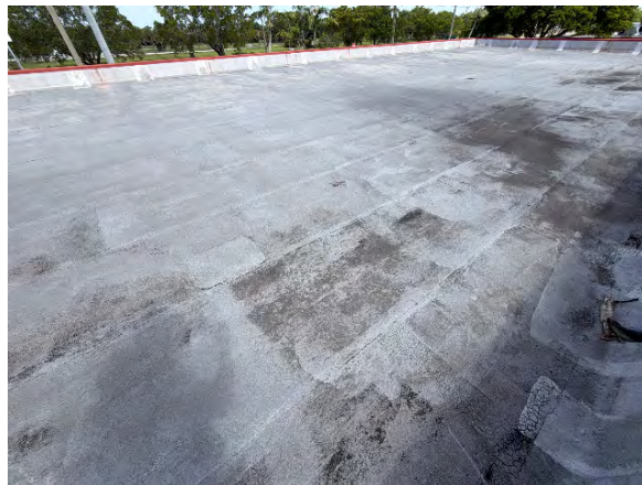
Roof overview facing west
