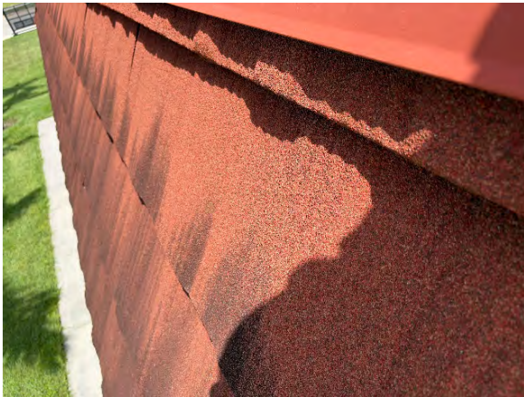
Metal mansard overview
