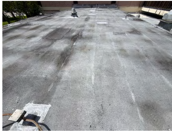
Roof overview facing south
