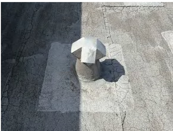
Typical roof vent with flashing detail
