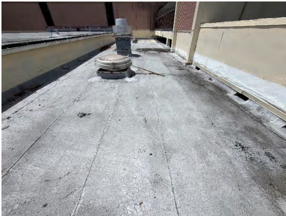
Roof overview facing south
