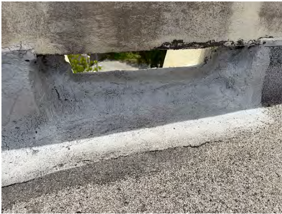
Typical overflow with flashing detail
