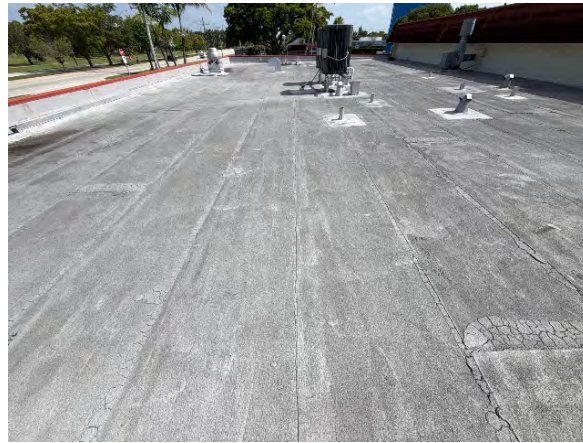
Roof overview facing north
