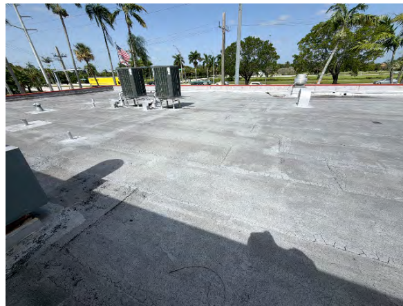
Roof overview facing west
