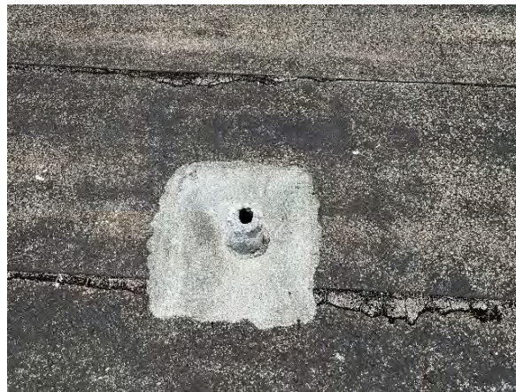
Typical plumbing stack with flashing detail
