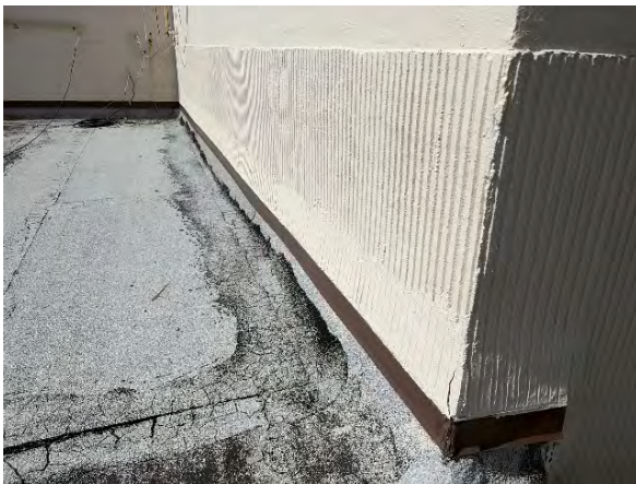
Typical counter flashing
