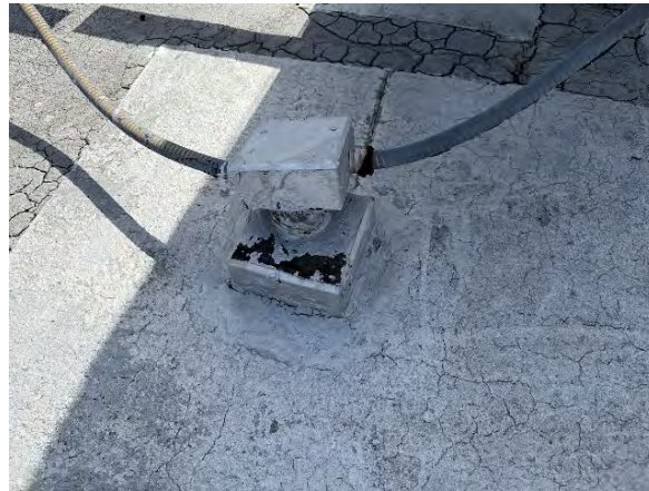
Typical pitch pan flashing detail
