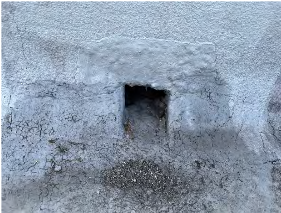
Typical primary scupper with flashing detail
