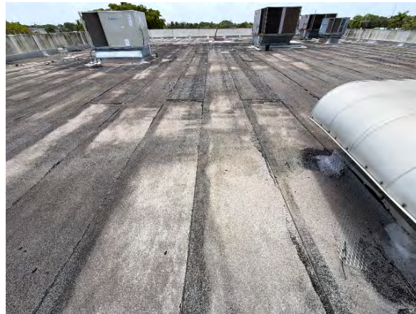
Roof overview facing west
