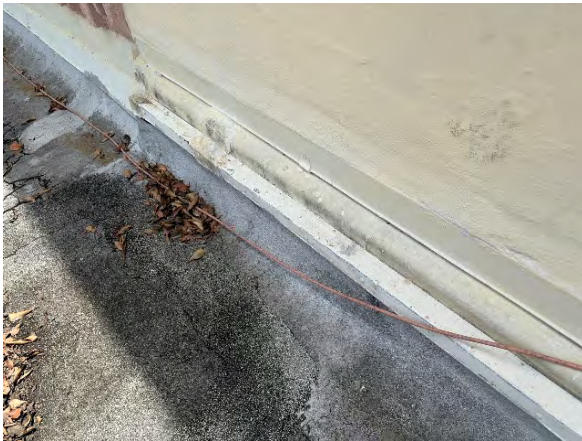
Typical expansion joint
