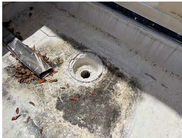
Typical roof drain with flashing detail
