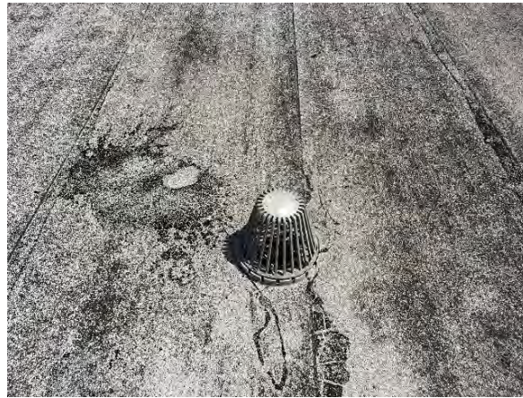
Typical retrofit drain
