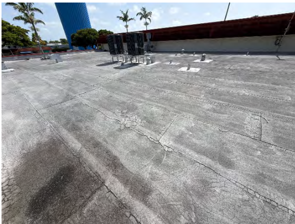
Roof overview facing east
