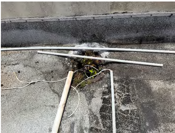
Typical roof drain with flashing detail
