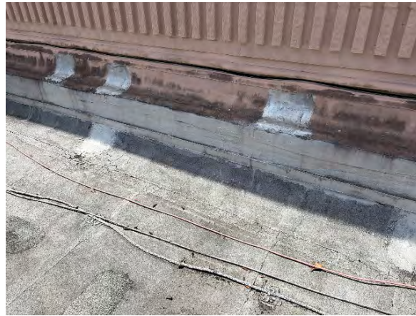
Typical expansion joint
