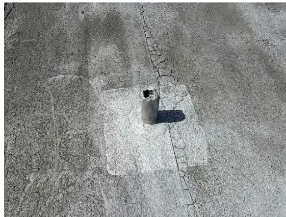
Typical plumbing stack with flashing detail
