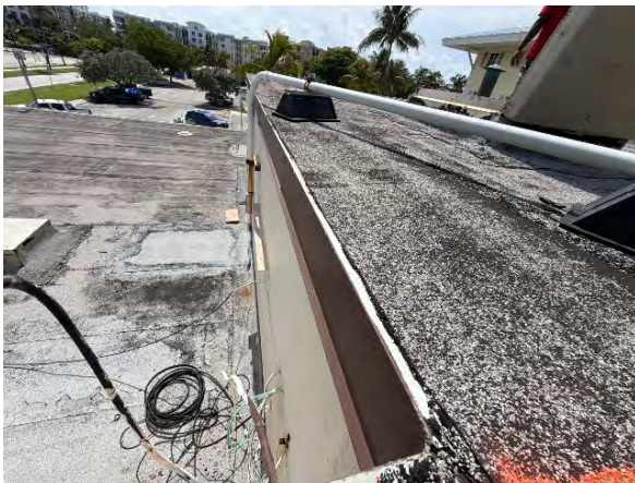
Typical drip edge with flashing detail
