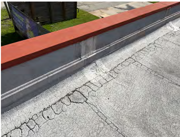
Typical parapet wall with base flashing detail
