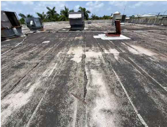
Roof overview facing east
