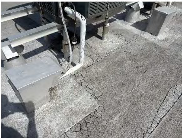
Typical line jack with flashing detail
