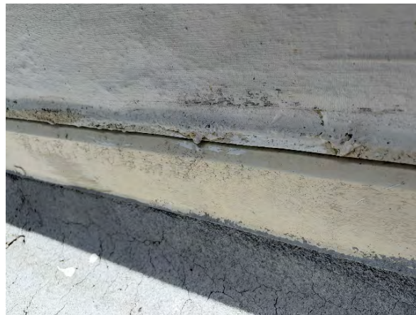
Typical stucco stop counter flashing
