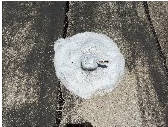
Typical pitch pan flashing detail
