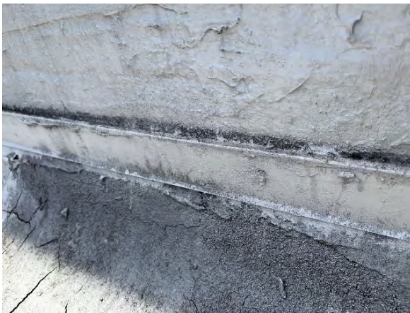
Typical stucco stop counter flashing
