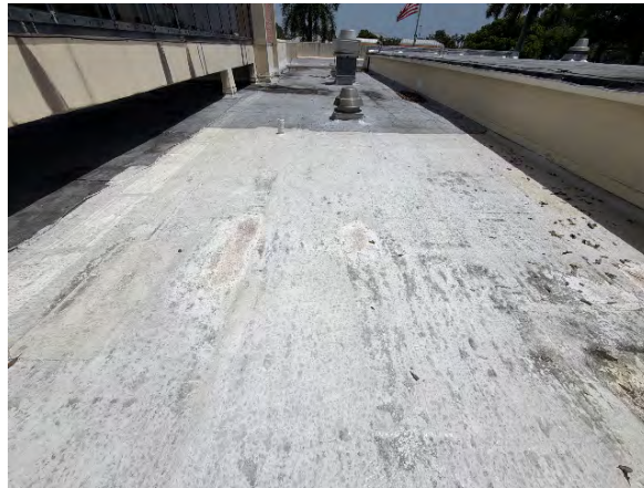
Roof overview facing north
