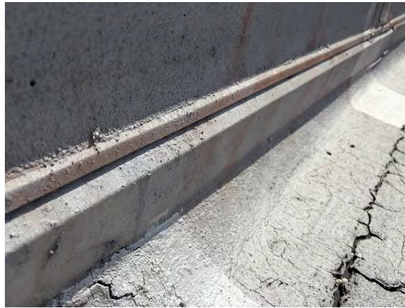
Typical surface mount counter flashing
