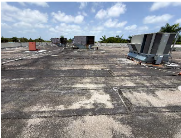
Roof overview facing north
