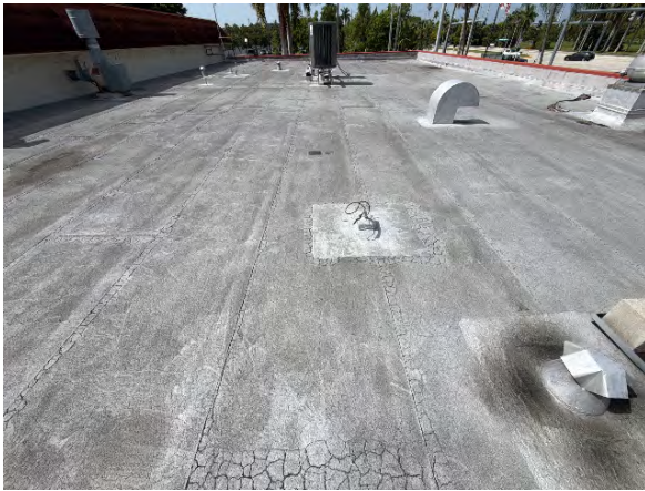
Roof overview facing south
