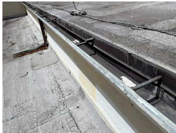
Typical gutter system with downspouts
