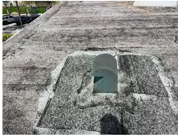
Typical gooseneck with flashing detail
