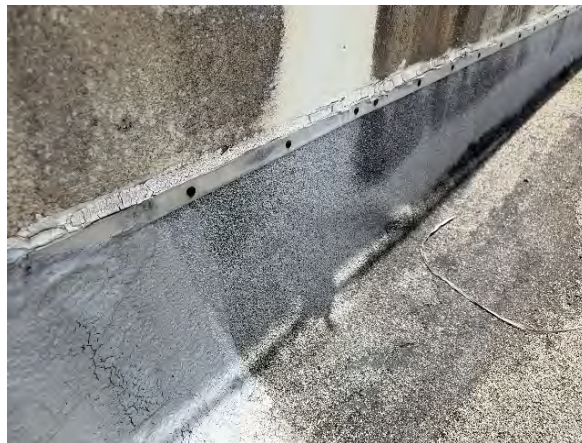
Typical termination bar counter flashing
