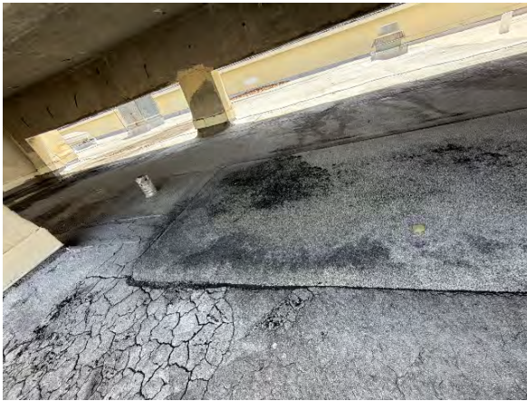
Roof overview facing east
