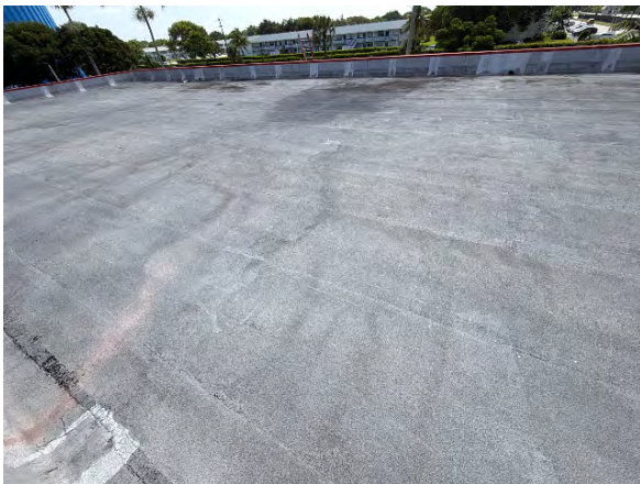
Roof overview facing east
