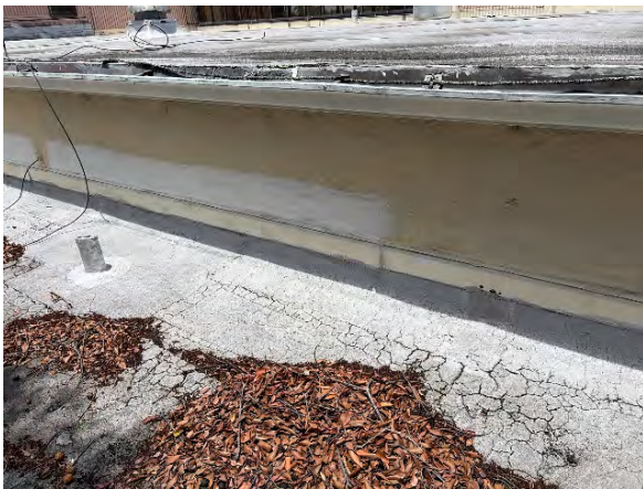
Typical wall with base flashing detail
