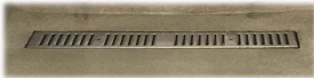
Figure 22 - Drain and Non-Porous Flooring in Each Kennel
