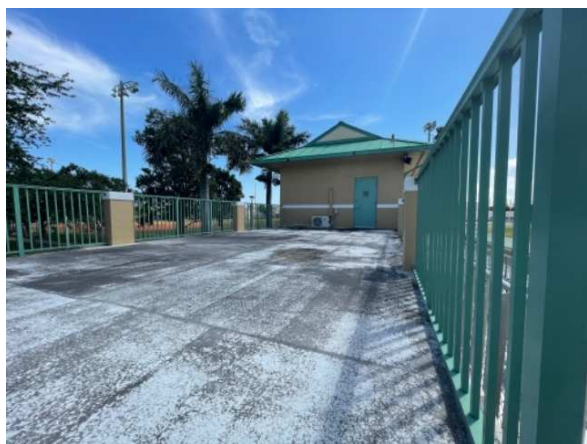
Overview of lower concrete section.
