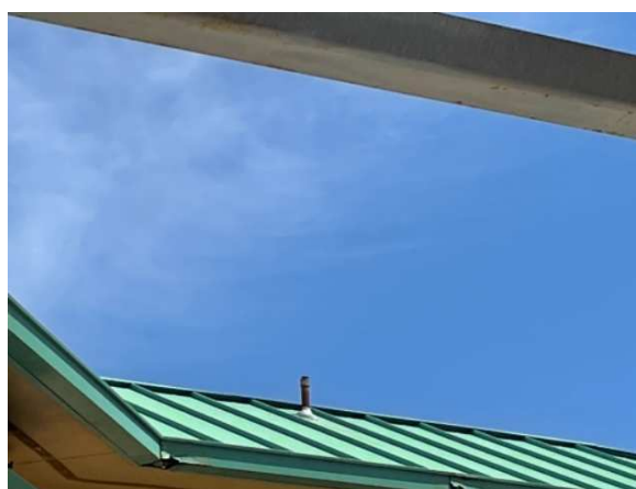
Typical plumbing stack with flashing detail.
