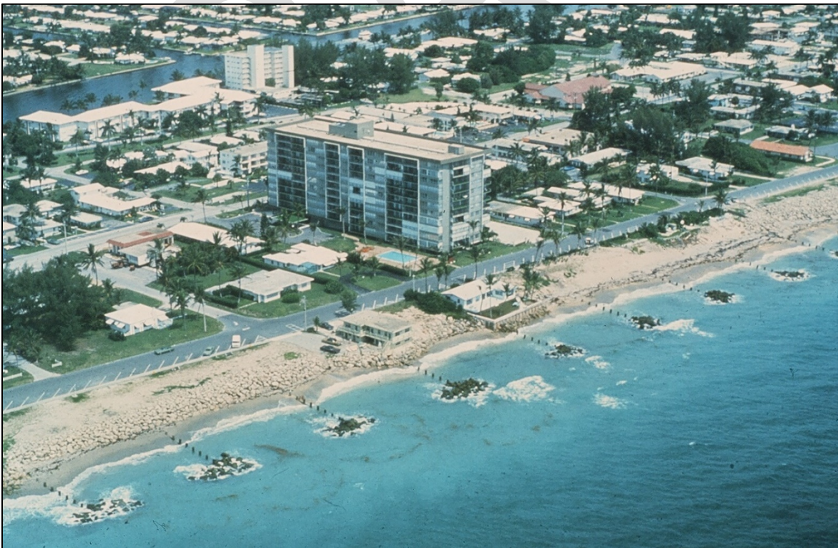
Figure 1: Rubble Mound Revetment circa 1974.
