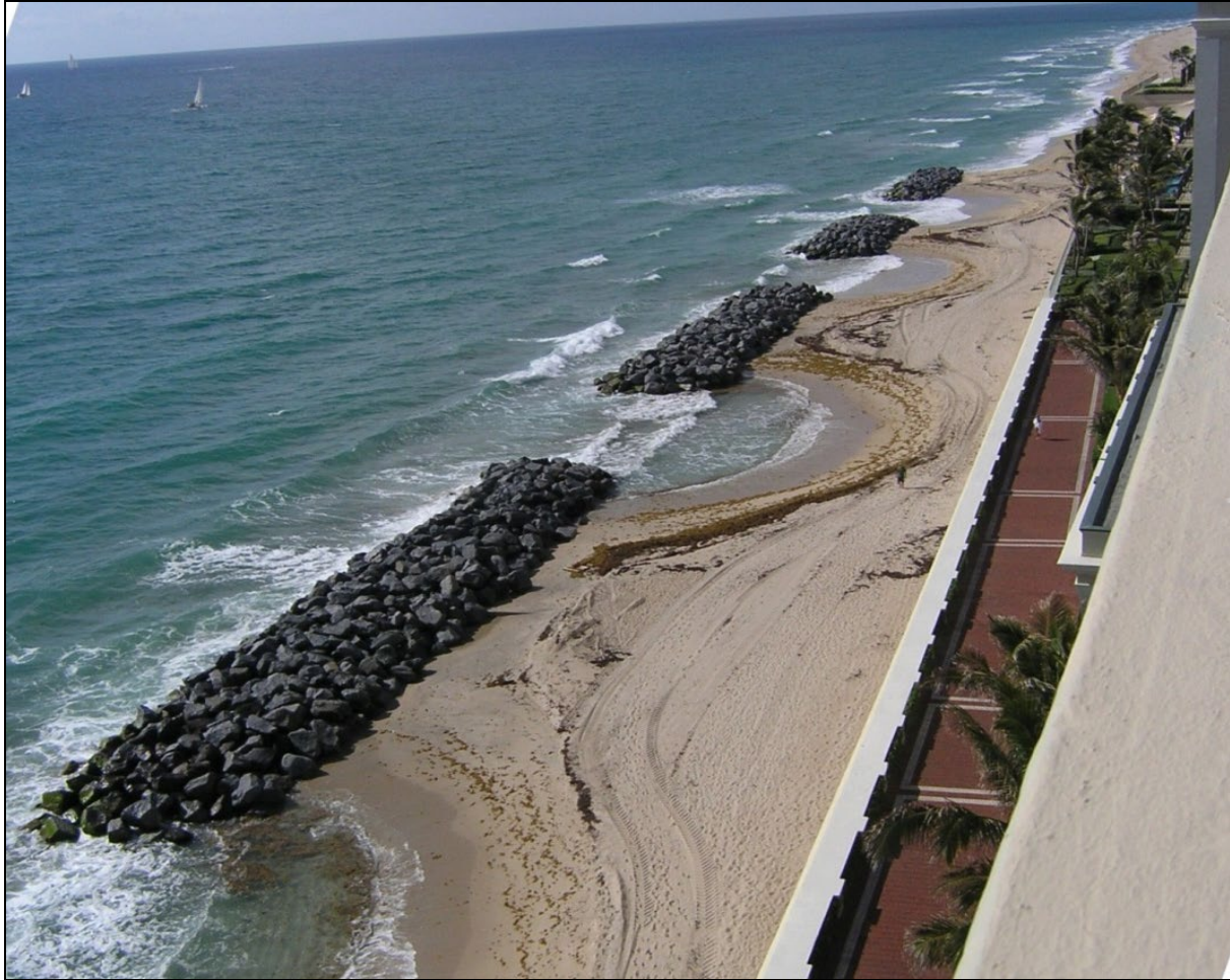
Figure 3: Rubblemound breakwaters (Town of Palm Beach).
