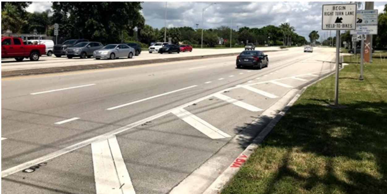
Figure 13: Powerline Road - Hillsboro Intersection, North Bound
