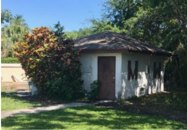
Figure 15: Restroom structure at River Park.
