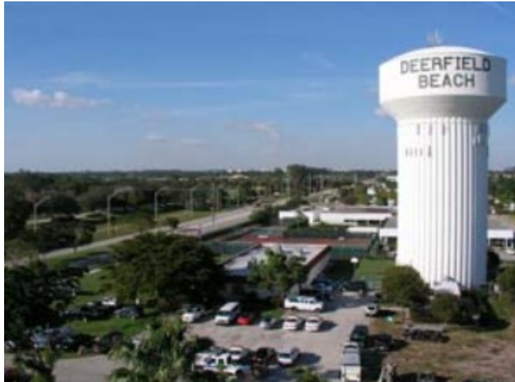
Figure 7: Deerfield Beach Water Tower
