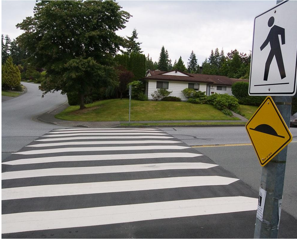
Figure 34: Raised crossing with signage
